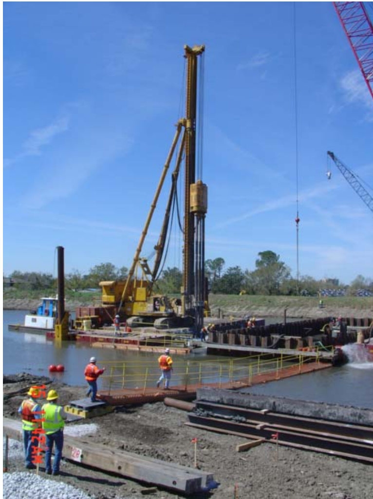
Figure 7. DMM machine (triple axis) operating in river conditions (Courtesy of Raito Inc.).
