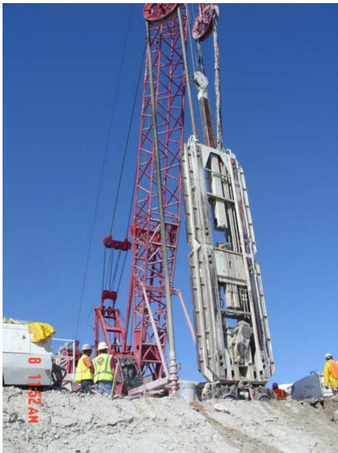
Figure 2. Hydromill being extracted from trench, at Herbert Hoover Dike, Florida (Courtesy of TreviCOS South).
