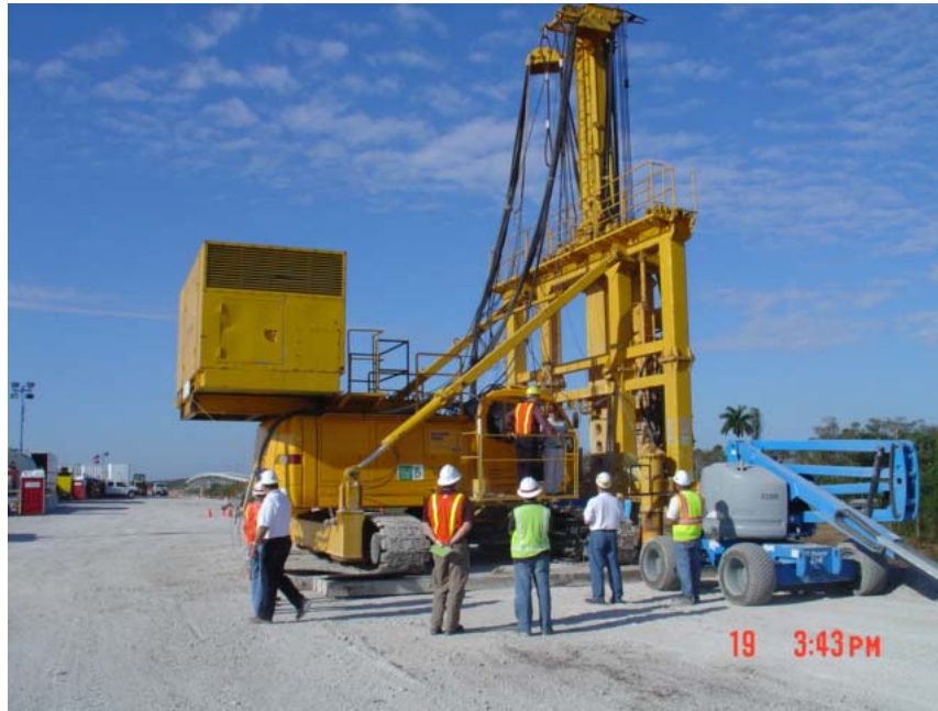
Figure 9. The TRD base machine, with the cutting post inserted into the ground. (Courtesy of Hayward Baker, Inc.)
