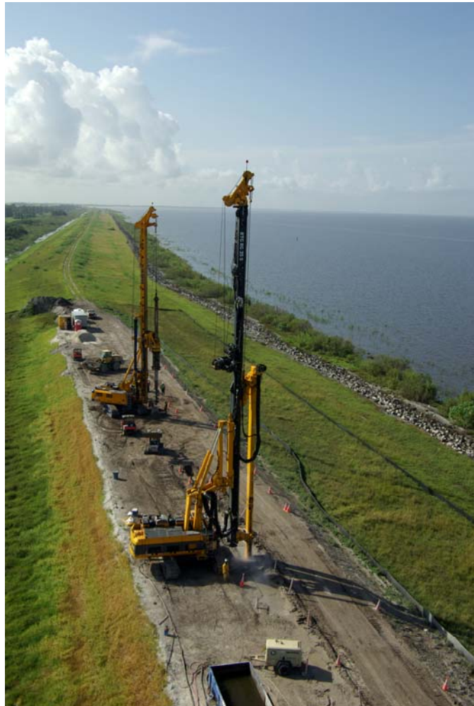
Figure 12. CSM machine (foreground) with predrilling being conducted in the background. (Photograph courtesy of Bauer Construction)
