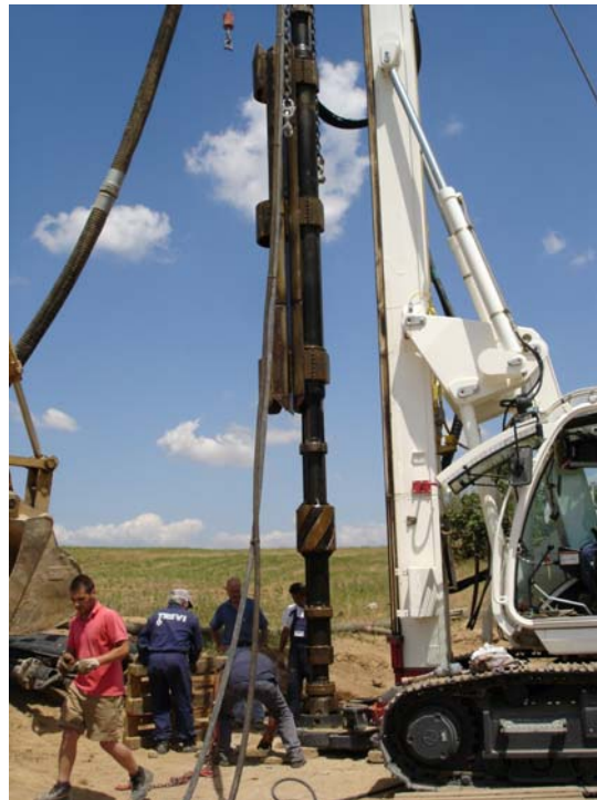
Figure 4. “Slot” being created by overlapping secant piles drilled consecutively.
